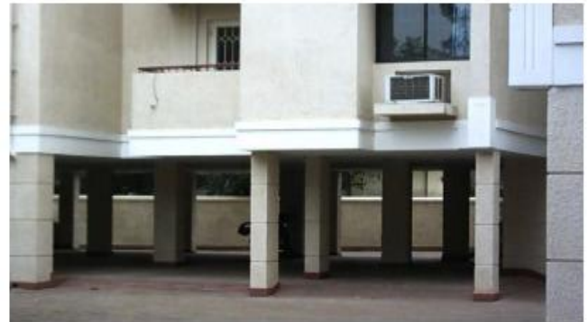
Fig. 1. Typical example of OGS building.
